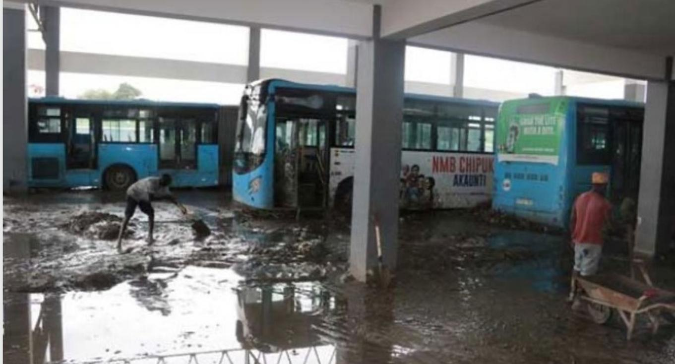
Source: Citizen Tanzania (2018). The Dar Es Salaam BRT depot was built in an area prone to flooding after BRT drivers and mechanics were ignored in an environmental assessment, with serious and ongoing ramifications (Stiller et al, 2019).
